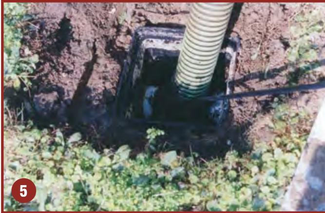
5 Be sure to inspect all connecting junction box locations (level, repair and adjust distribution flow), then jet junction boxes and drop boxes (to achieve adequate flow and distribution of materials during remediation, and following the treatment process).
