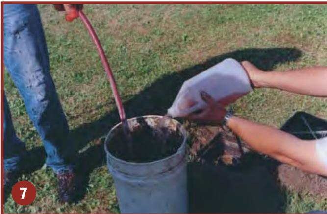
7 Blend each **PRO-PUMP** material with tap water prior to addition to the system.
