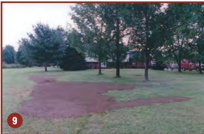
9 Inspect and review the absorption field area for possible drainage problems and make sure the absorption field is secure from water run-off. If necessary construct a curtain drain to divert flow away from the absorption area.
