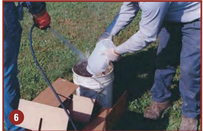
6 Following system preparation, prepare **PRO-PUMP® Bio-remediation** materials by pre-mixing each **PRO-PUMP** formulation with 3 to 5 gallons of tap water, then distribute equally to each of the system lines.
