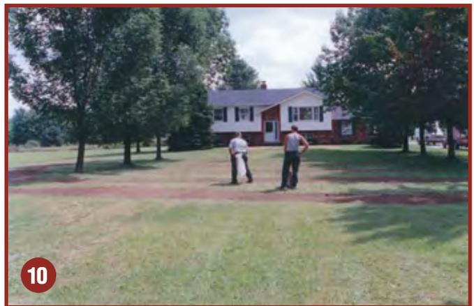
10 On completion of the bio-remediation process, check the field grade and fill any low spots where the absorption filled lines run. This will eliminate unnecessary water collection above and within the absorption area. ***Your customers will love the technology, results and cost savings!***
