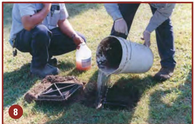
8 Following dilution with tap water add the **PRO-PUMP** formulations directly to the absorption systems via the systems junction box.
